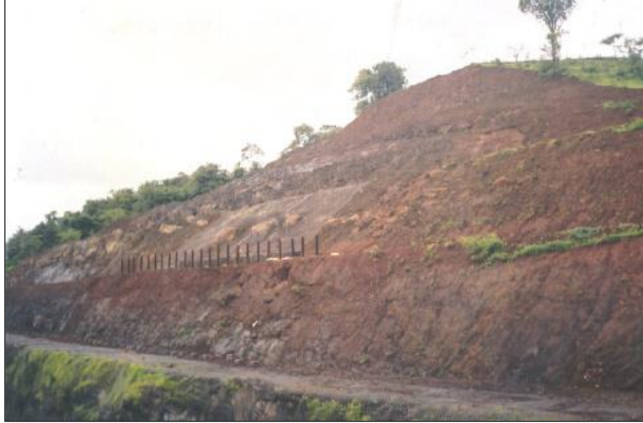
RAJAPUR SOUTH FRACTURED ROCK CUTTING
