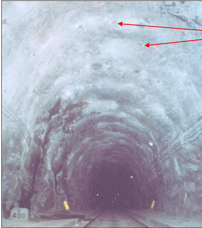
ROCK BOLTING IN KARBUDE TUNNEL
