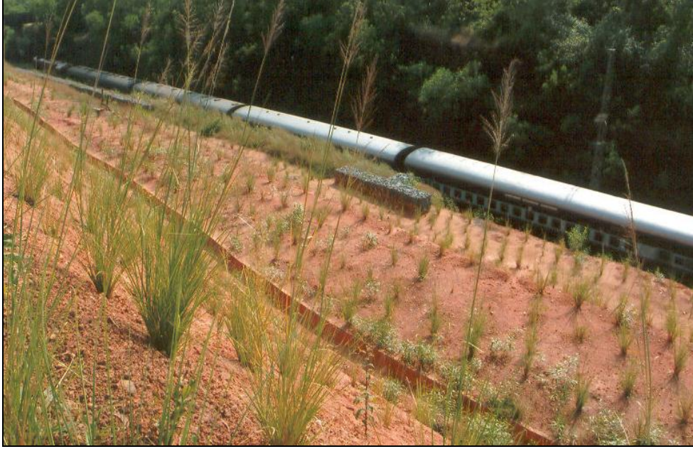
GRASS PLANTATION ON CUTTING SLOPE
