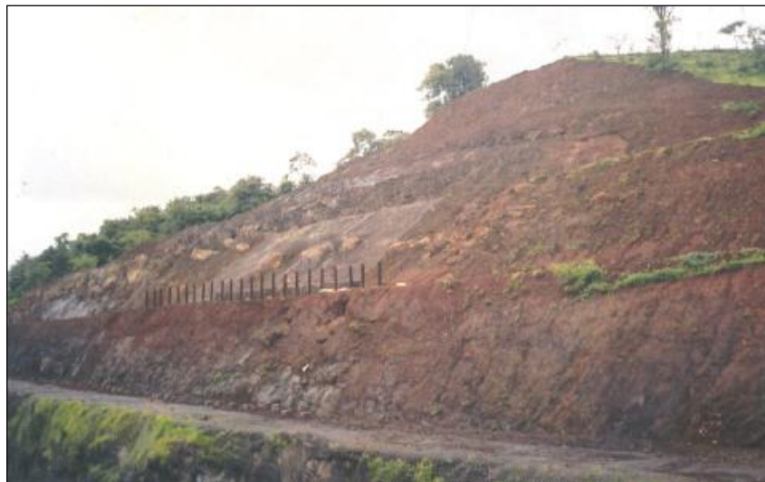
RAJAPUR SOUTH CUTTING
