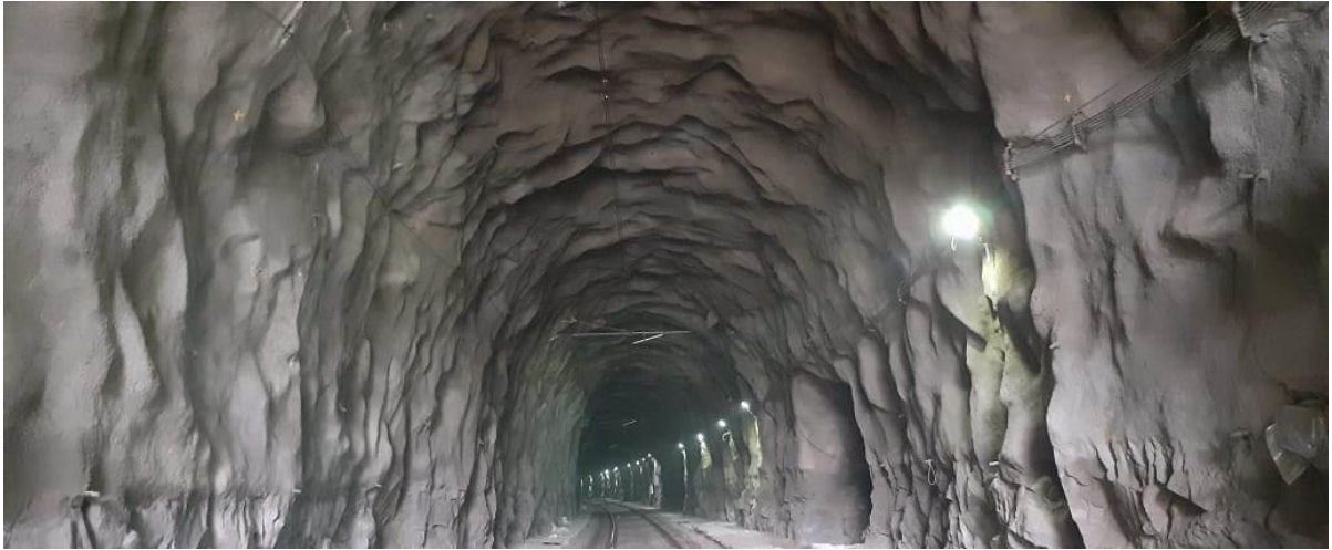
Rockbolting and Shotcreting at Ashti tunnel
