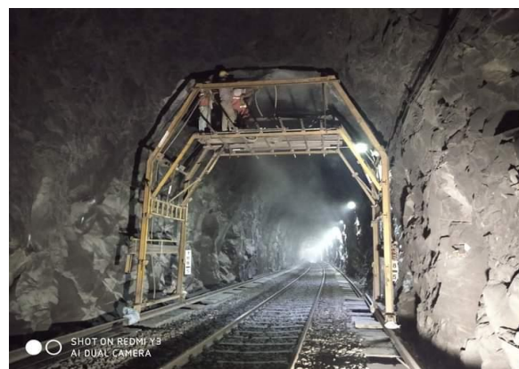
Shotcreting work at Ashti Tunnel
