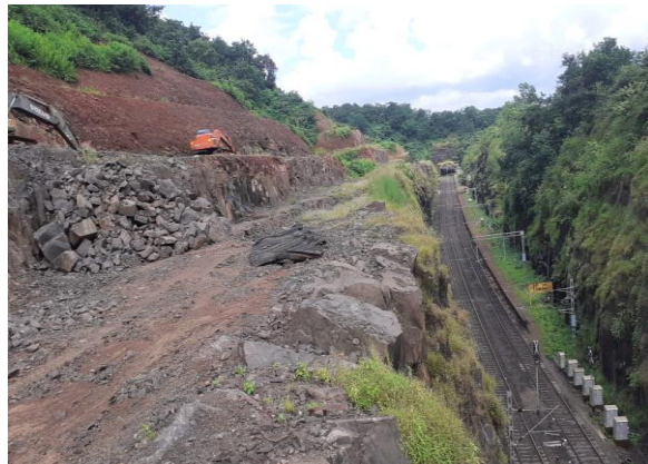
Hard rock cutting at Ukshi
