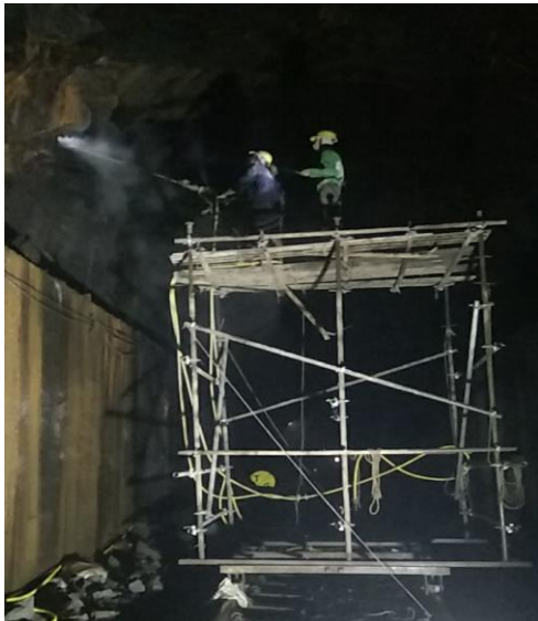
Rockbolting at Padi tunnel
