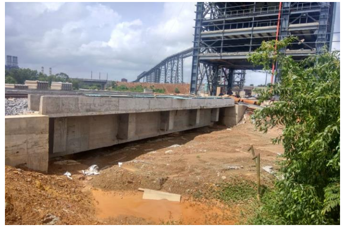
Bridges no 2 at Chainage-636.
