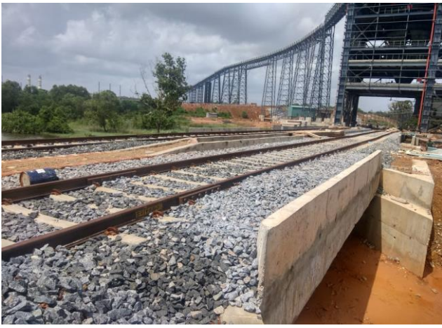
Bridge no 1 at Chainage-600
