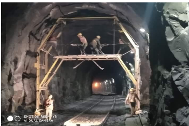
Rockbolting work at Ashti Tunnel
