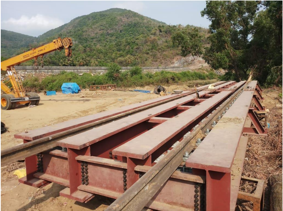
Assembling of RH Girder at Seabird RUB @ Km 512/210
