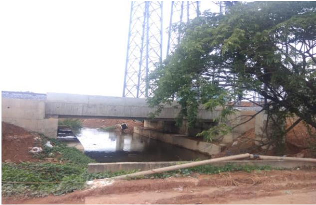
Bridge no 3 at Chainage-740
