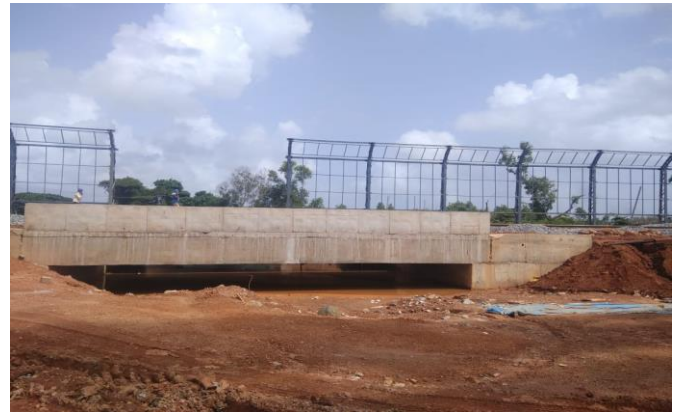
Bridge no 4 at Chainage-840
