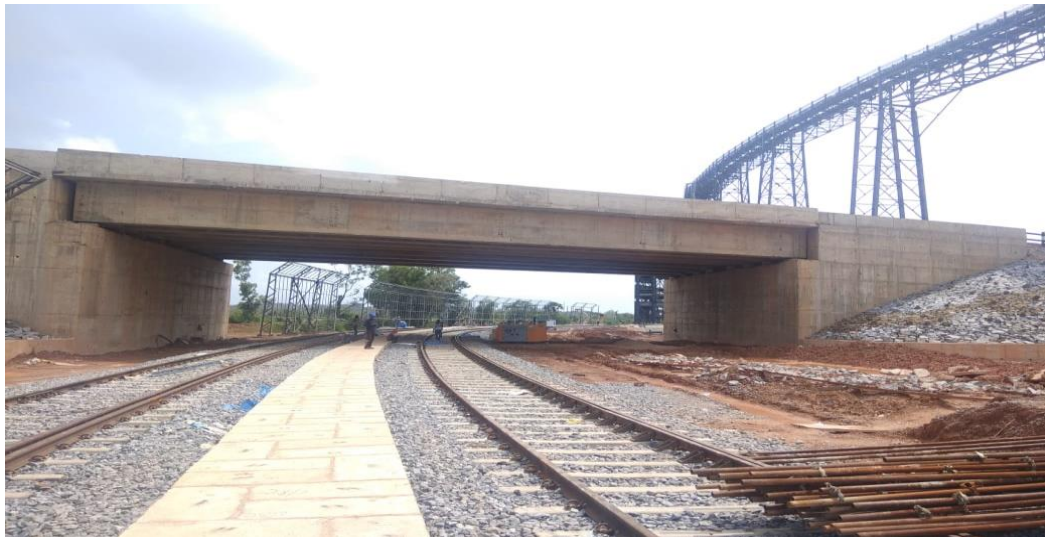
Bridge no 5&6 at Chainage-880/890
