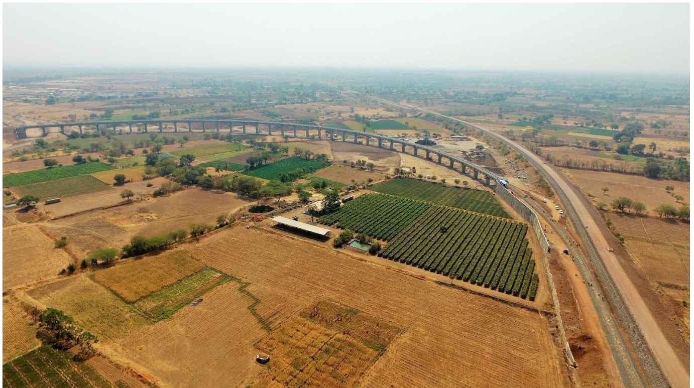
A view of NTPC Thermal Plant and 700m long Railway Viaduct constructed by KRCL in record six months time at Kudgi, Karnataka
