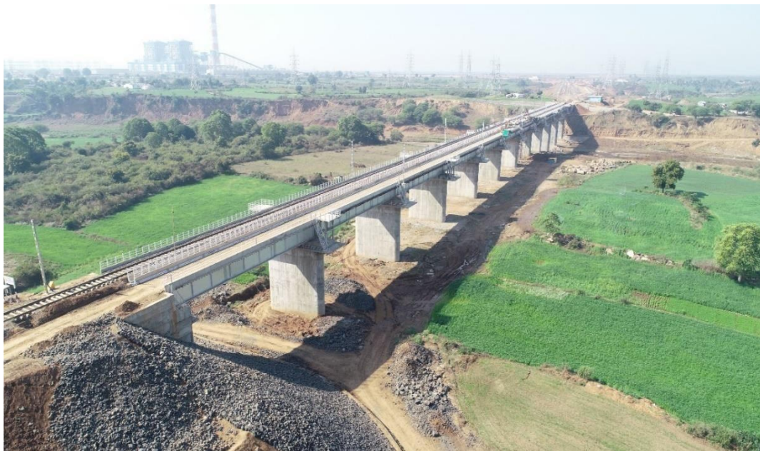
Br. No. 12 across Shakkar River at Km. 06/830 (12x30.5 m Composite Girder)
