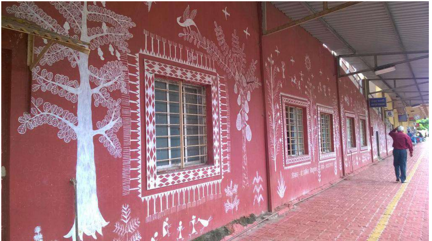
Paintings on Ratnagiri Station Building Walls
