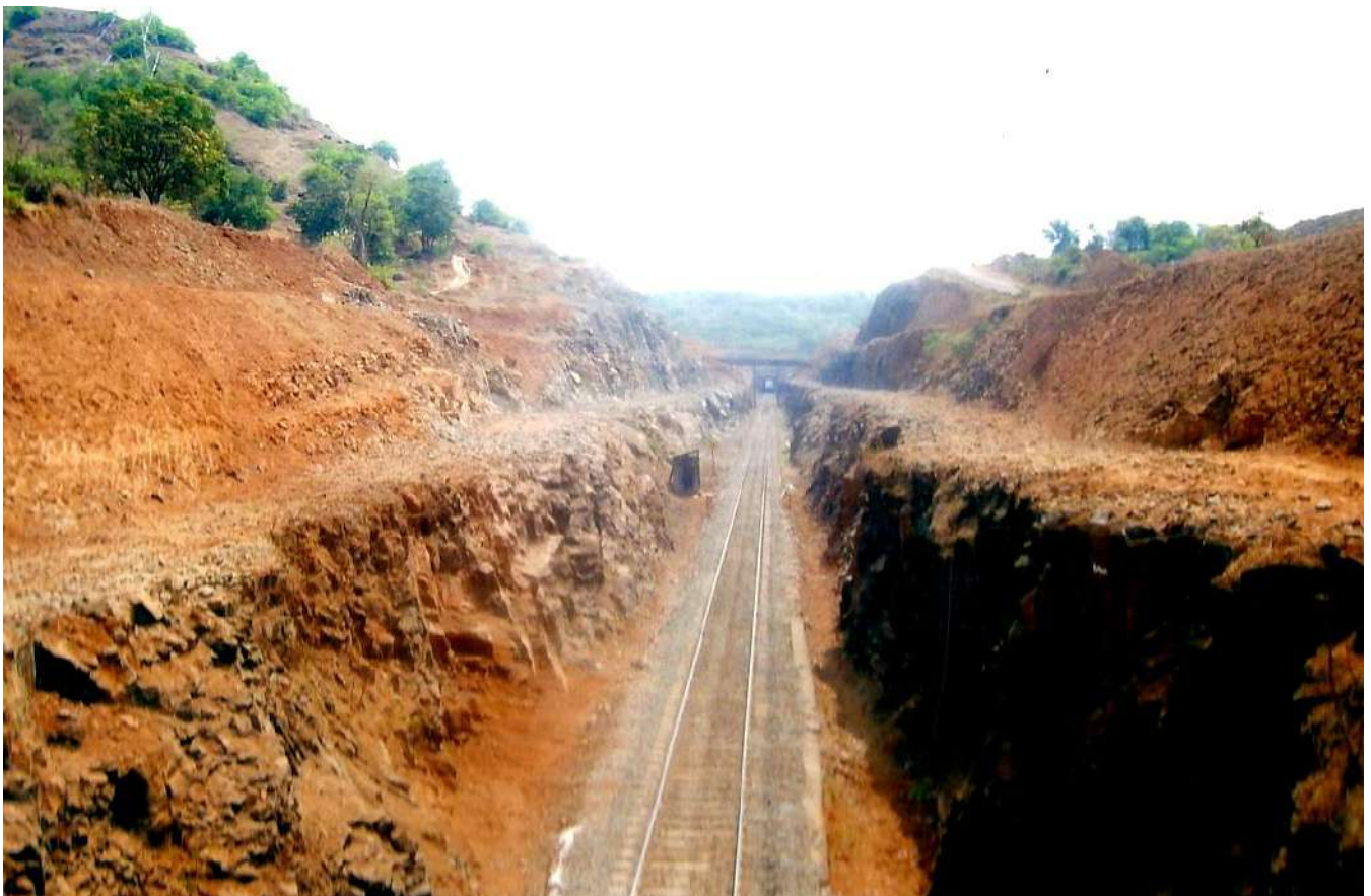
Slope Flattening Work at Rock Cutting (Before and After Safety Work)
