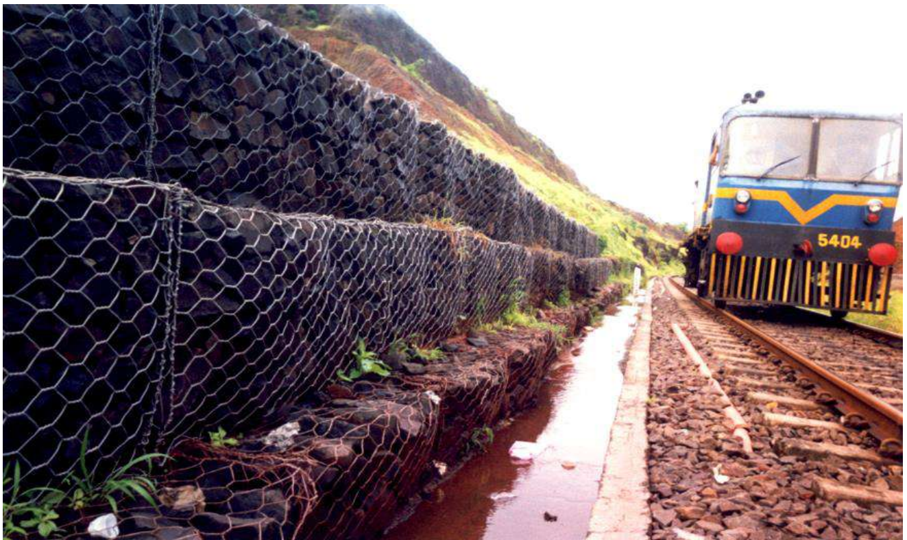
GABION RETAINING WALL
