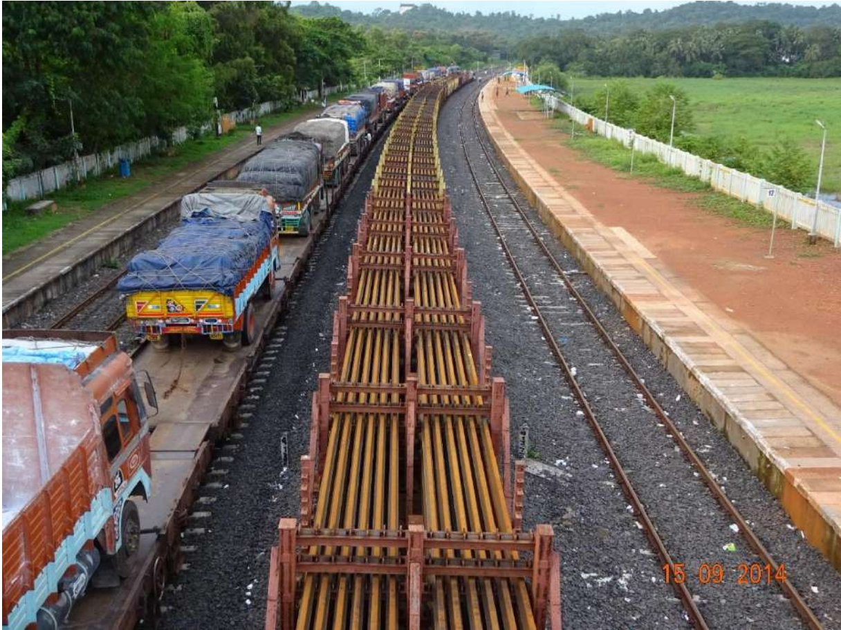
New 260m Rail Panels for Casual Rail Renewal
