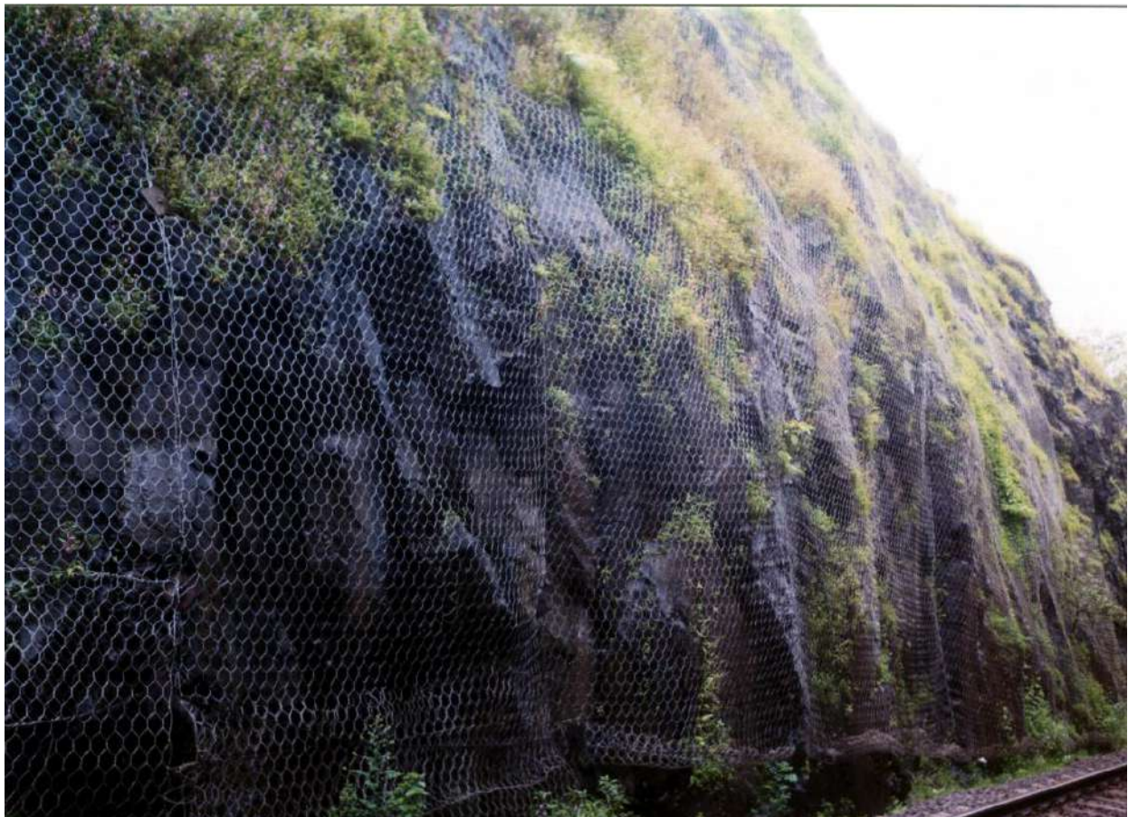
Medium Strength Boulder Net at Rock Cutting
