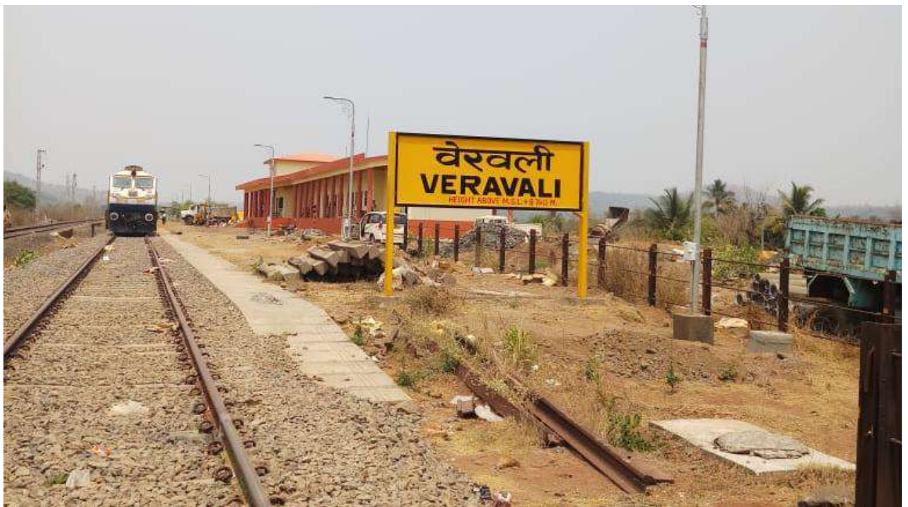
Creation of New Assets - Station at Veravali near Vilavade, Maharashtra
