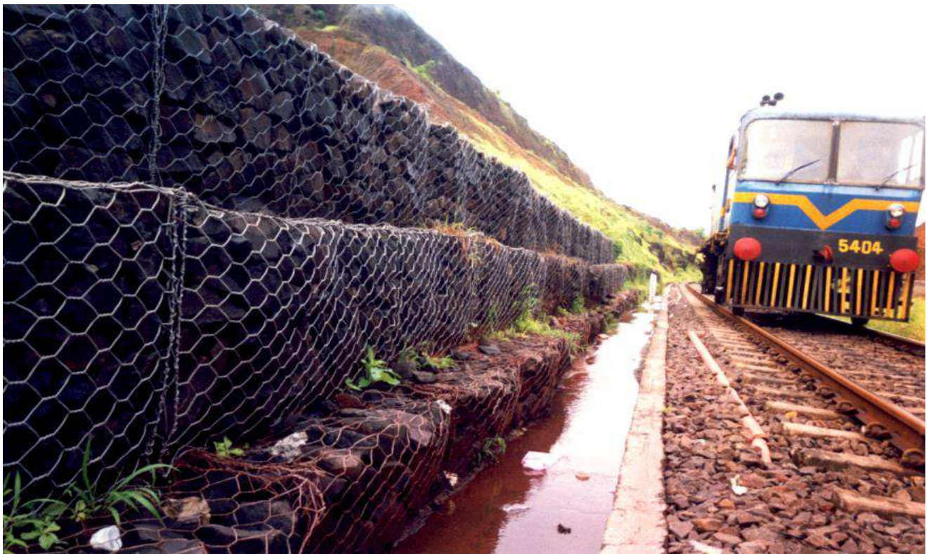
GABION RETAINING WALL
