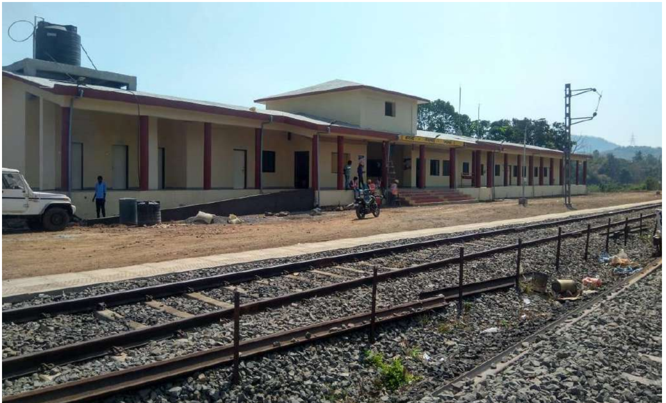
Creation of New Assets - Station at Kadavai near Sangmeshwar, Maharashtra
