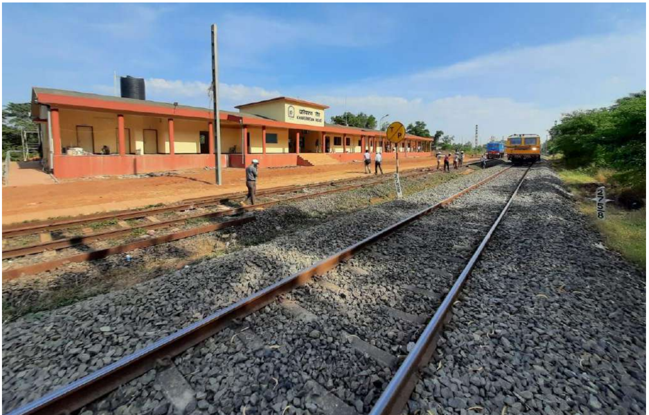
Creation of New Assets - Station at Kharepatan Road near Rajapur, Maharashtra
