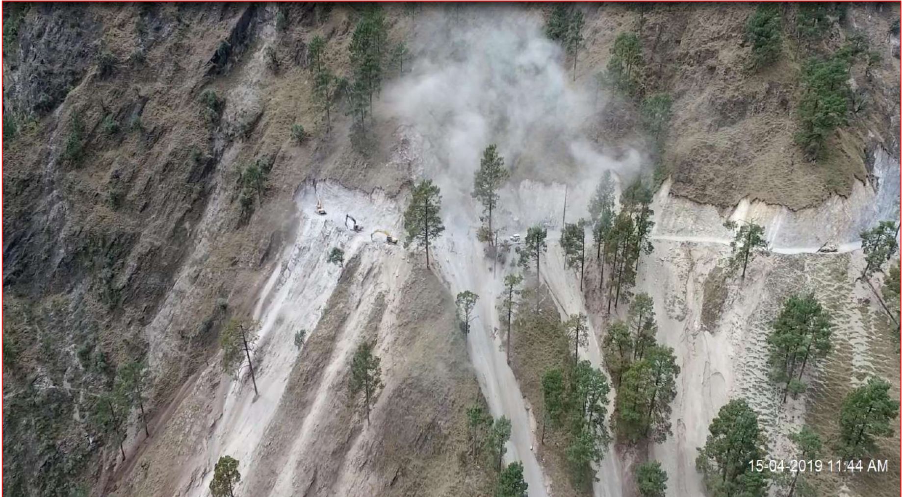
Ind-Adit T14 Approach Road
