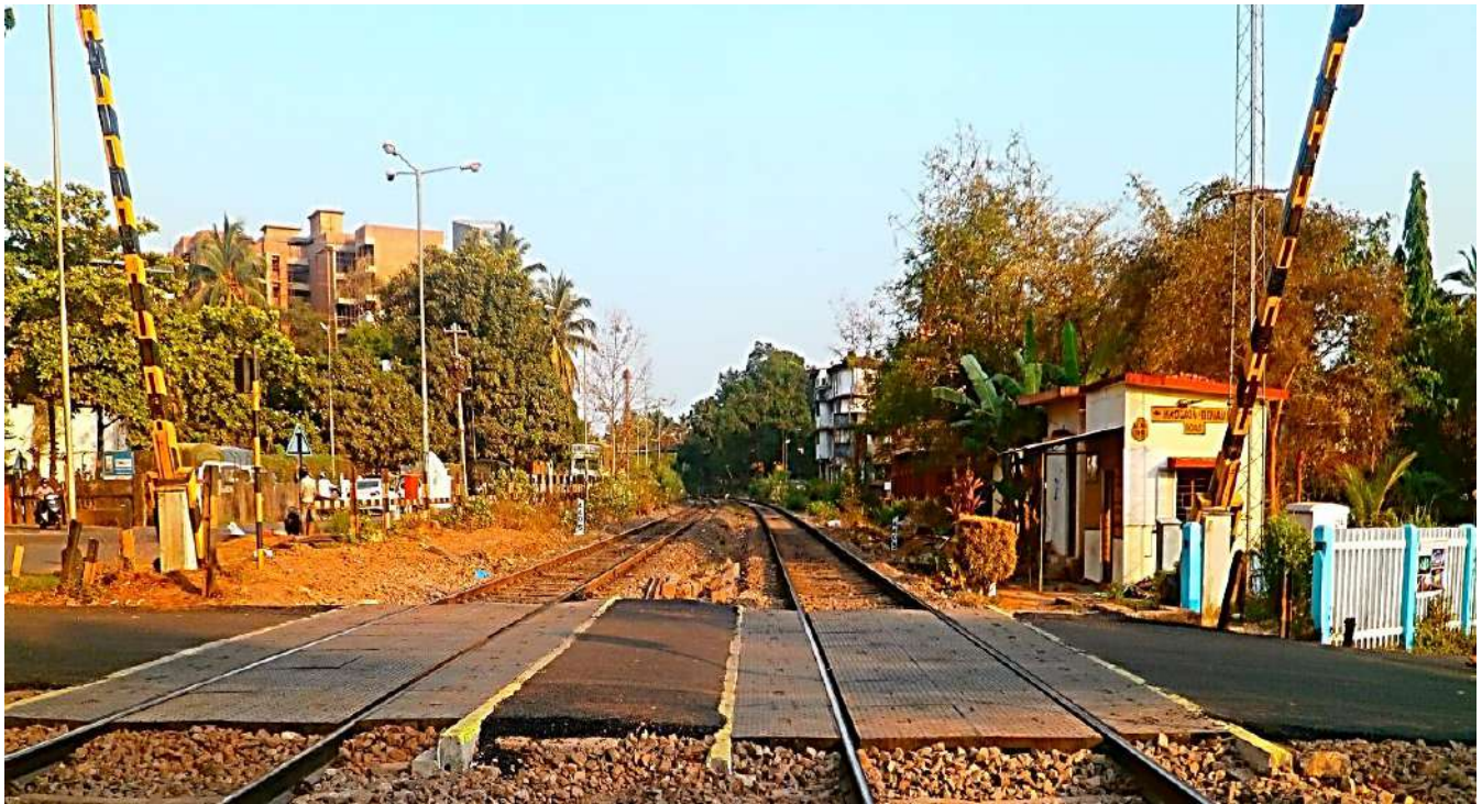
Rubberised Paver Blocks on Level Crossing Gate Road surface
