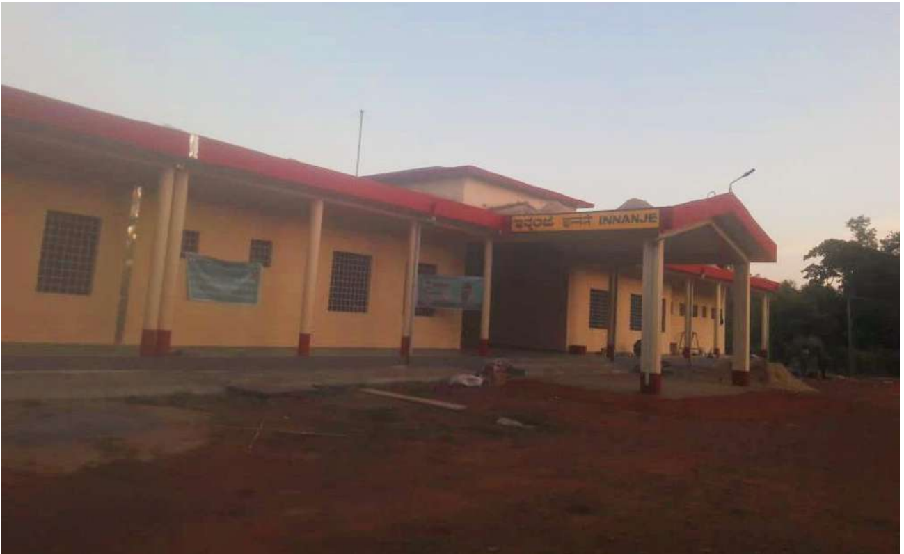
Creation of New Assets - Station at Innanje near Udupi, Karnataka
