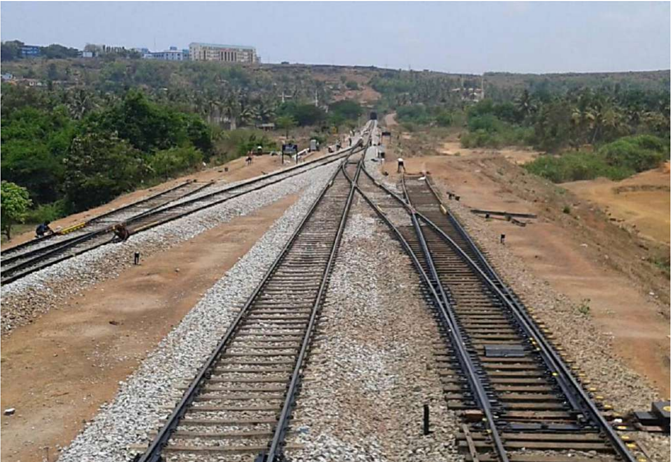
Thick Web Switches in Turn-outs
