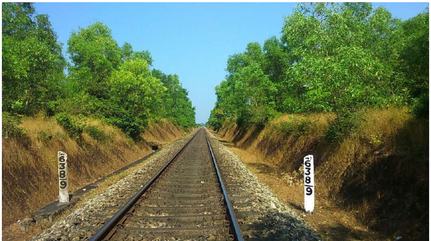
Green Railway – General view of Track
