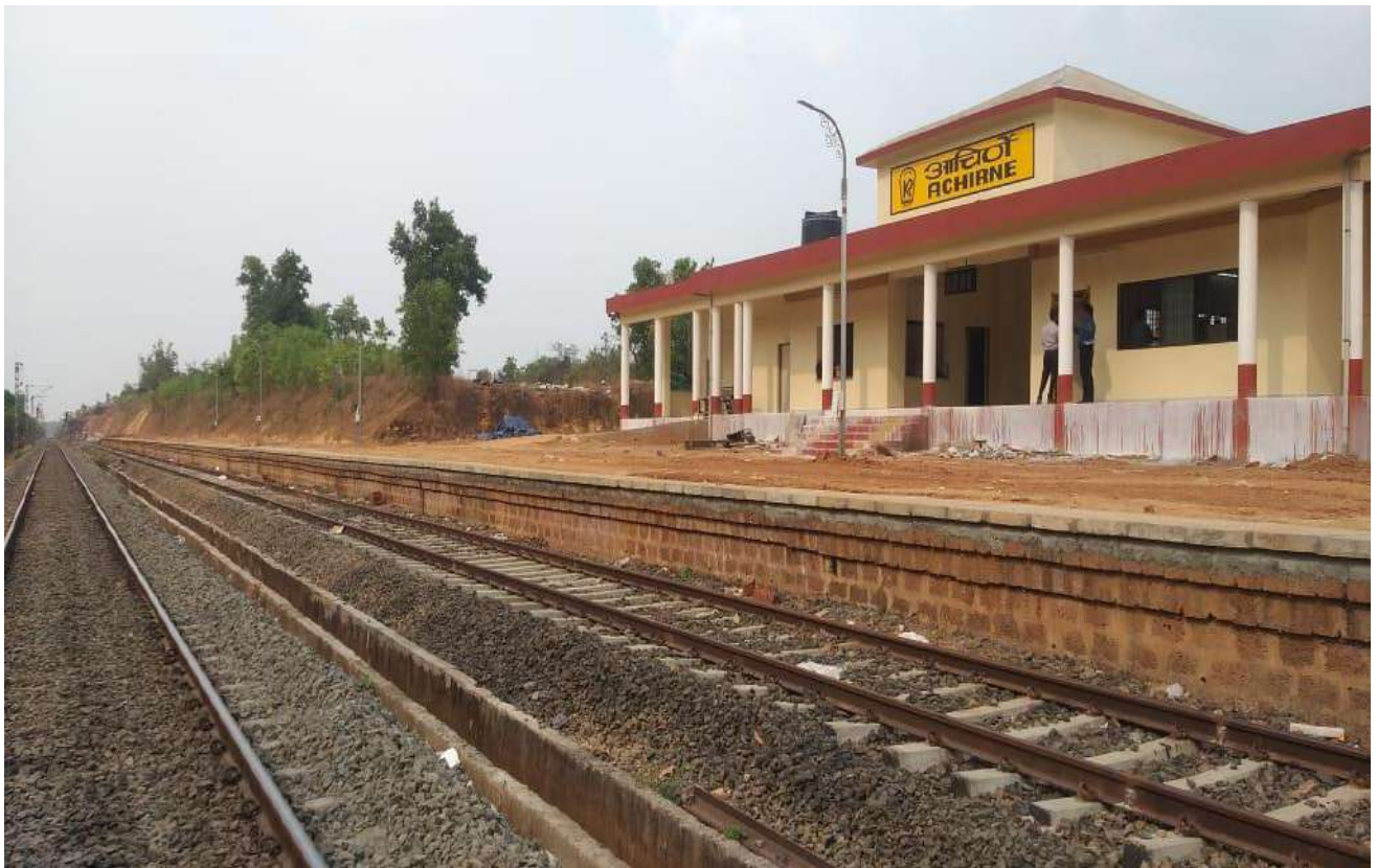
Creation of New Assets - Station at Achirne near Nandgaon Road, Maharashtra
