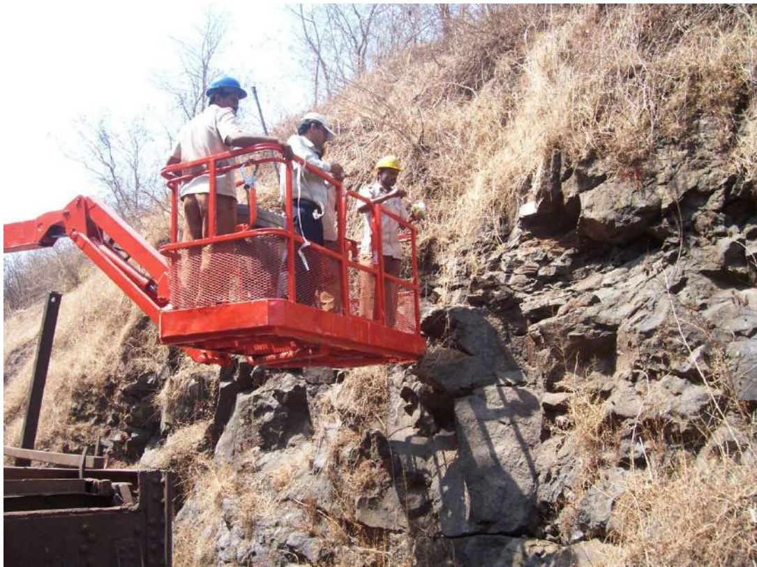
Inspection and Loose scaling in Rock Cuttings using Boom List
