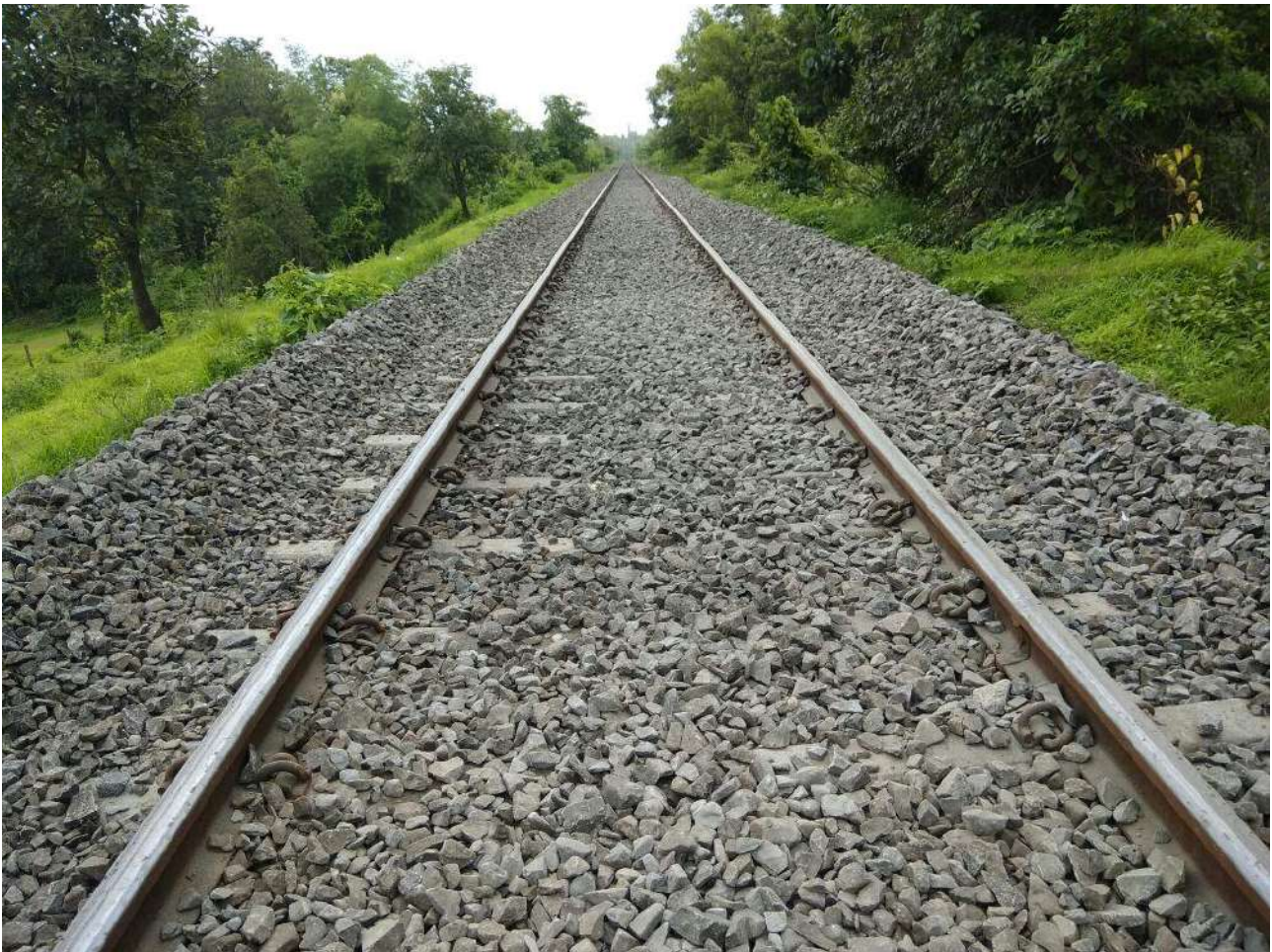
Working of Track Machines (Ballast Regulating Machine)
