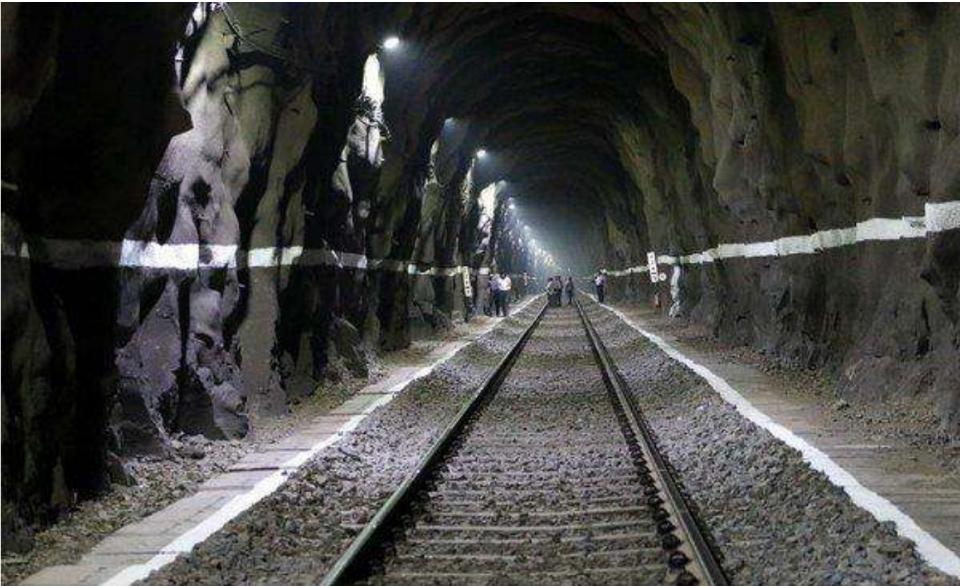
Permanent support in Tunnels - Rock bolts and Shotcreting
