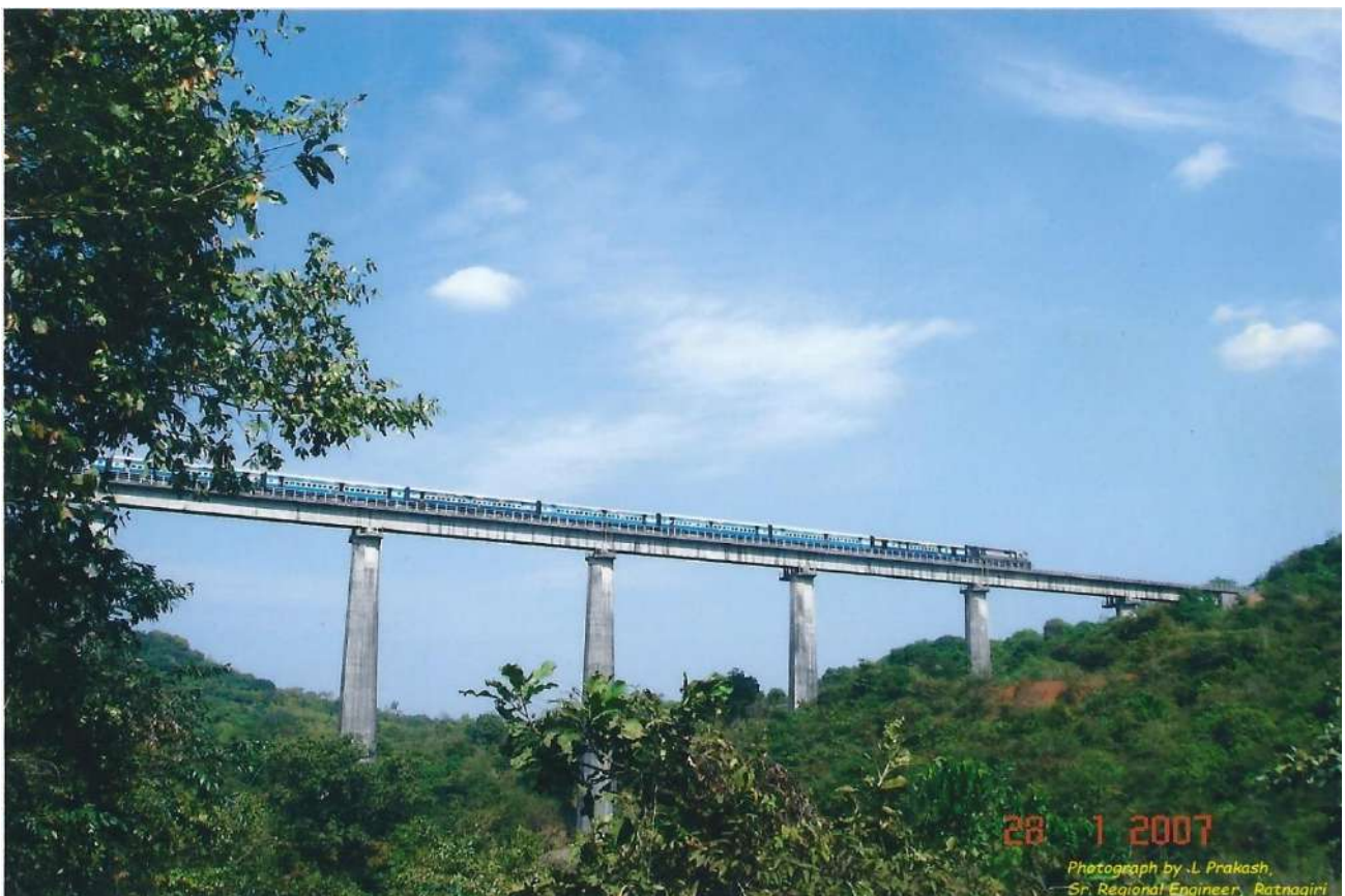
Panval Viaduct- Tallest Bridge on Konkan railway
