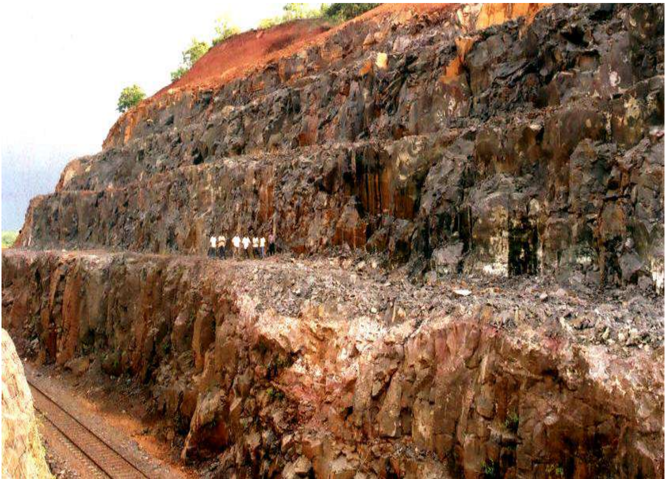
Slope Flattening Work at Rock Cutting (Before and After Safety Work)
