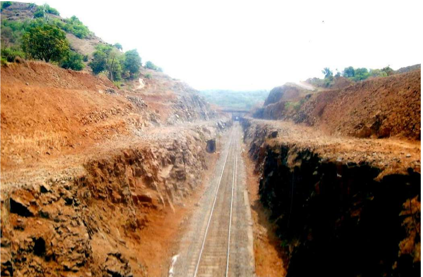
Slope Flattening Work at Rock Cutting (Before and After Safety Work)
