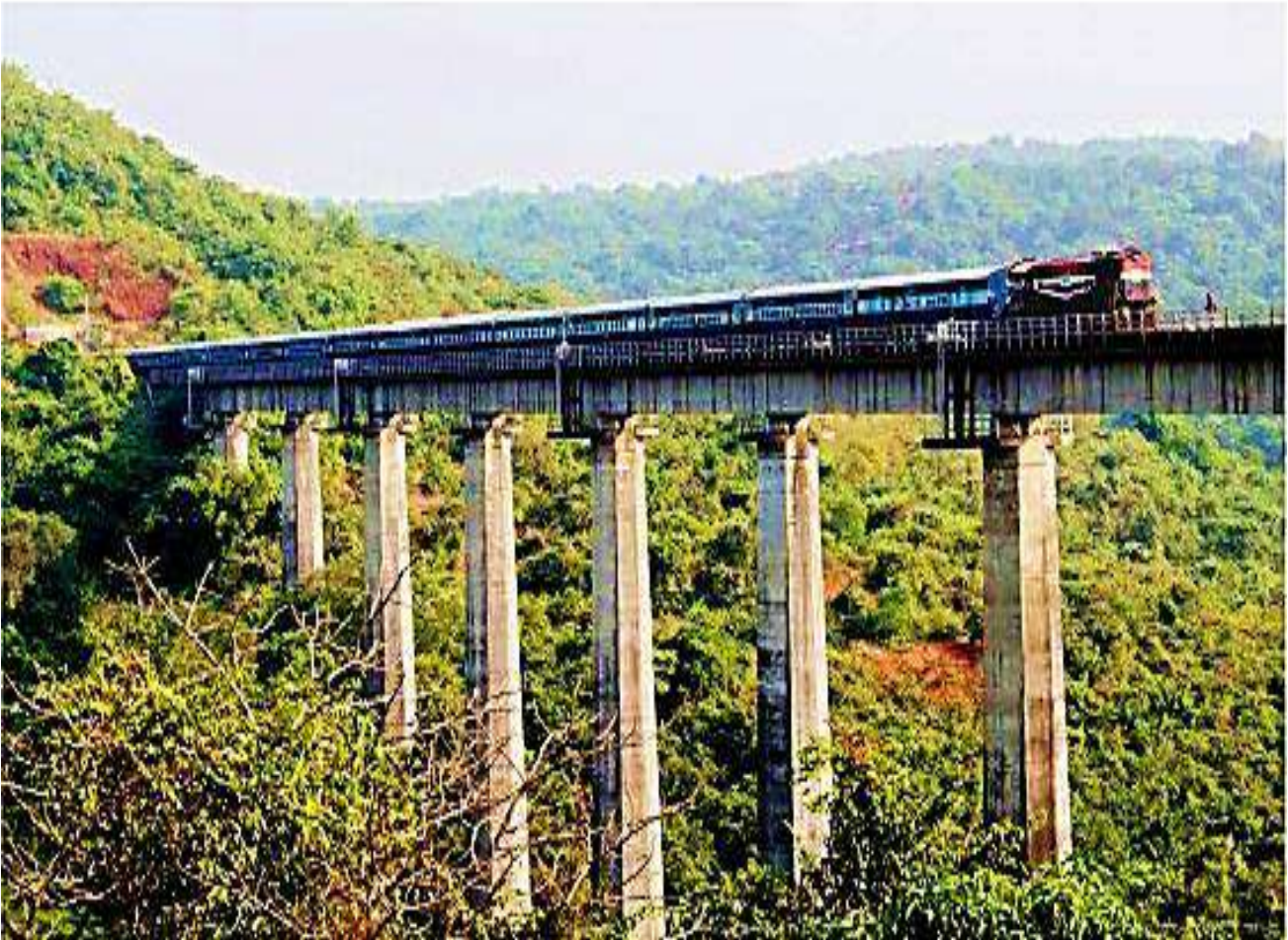
Panval Viaduct- Tallest Bridge on Konkan railway
