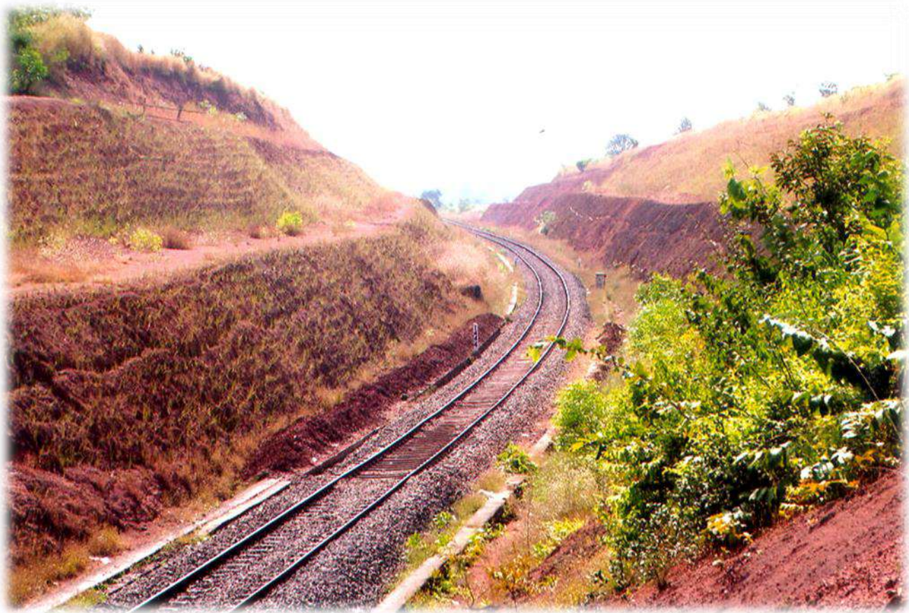
Vettiver Plantation on Soil Cutting Slopes for prevention of Soil erosion
