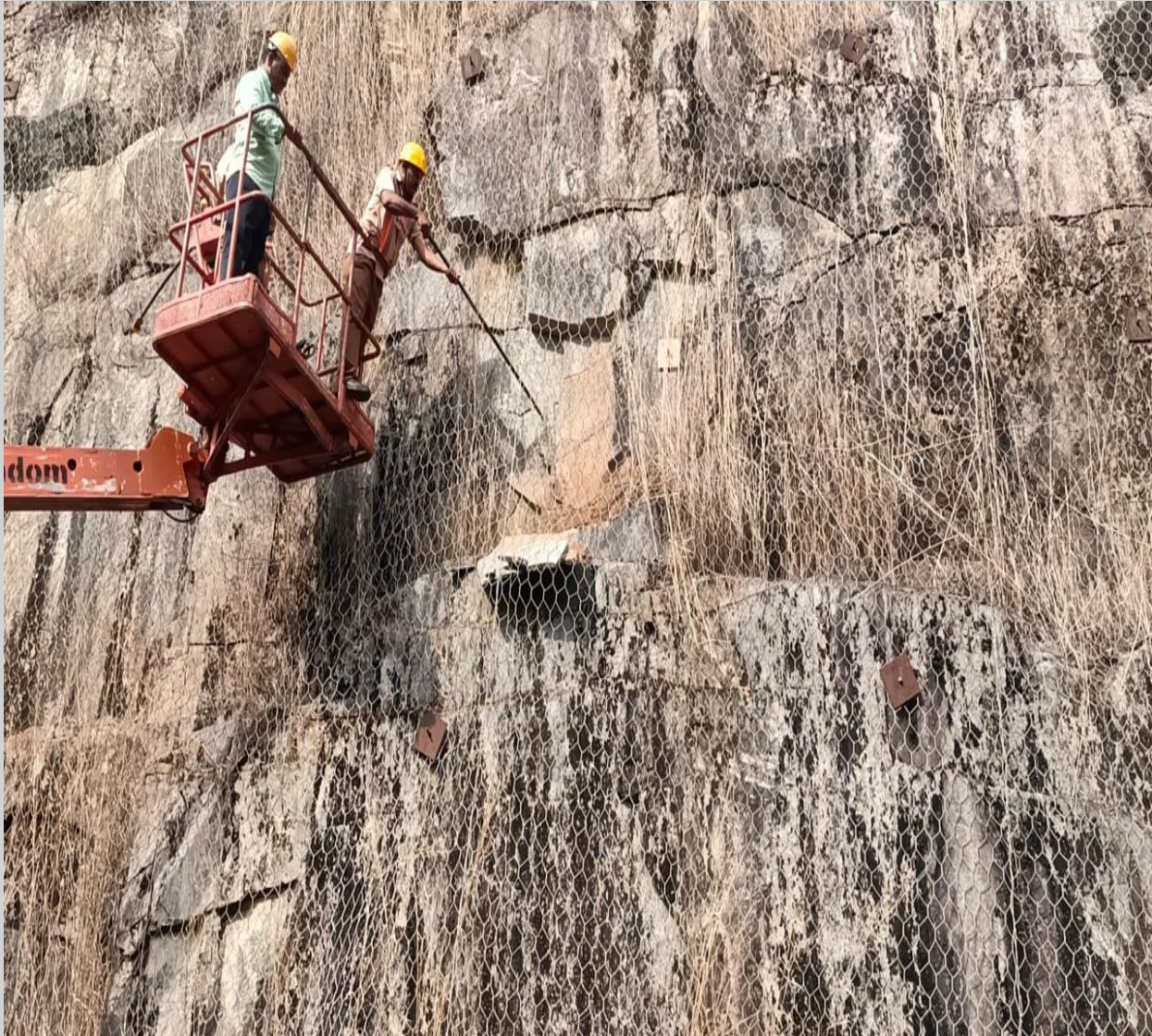
Inspection of High Depth Cuttings Through Boom Lift
