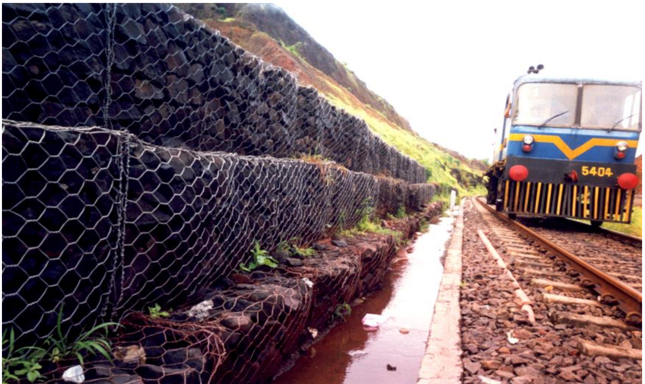
GABION RETAINING WALL
