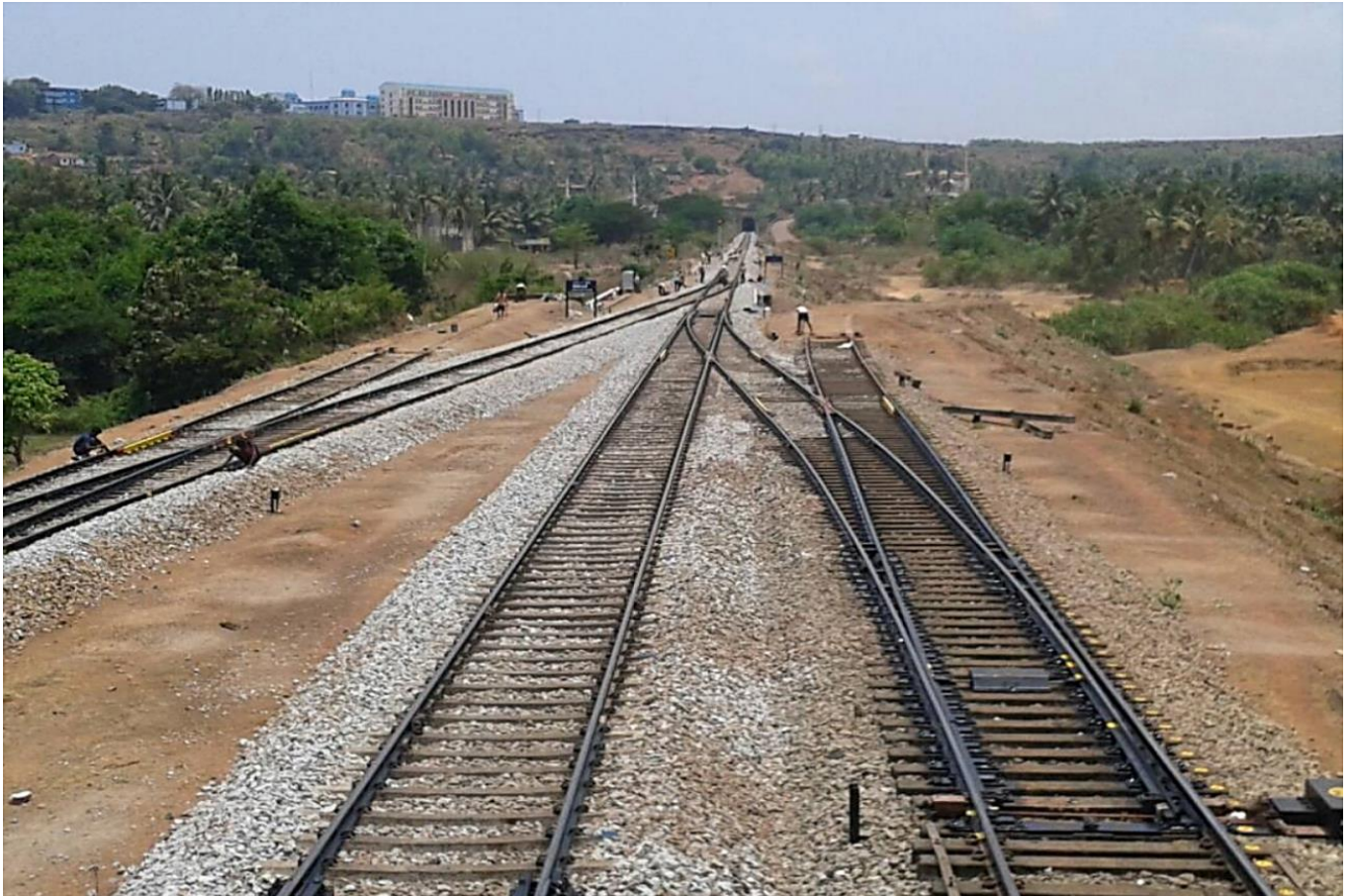
Thick Web Switches in Turn-outs
