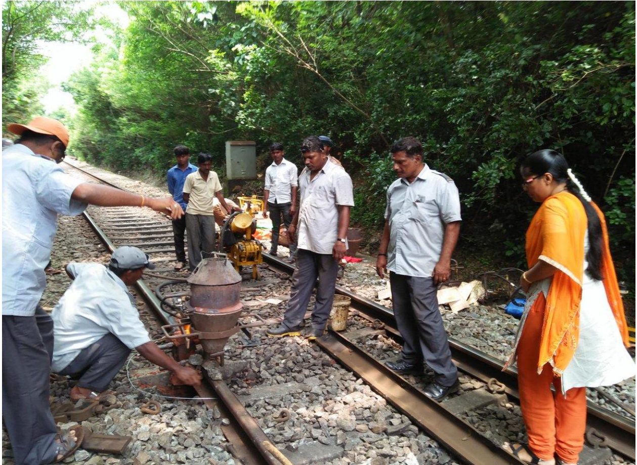
Alumino- Thermic Welding of Rails
