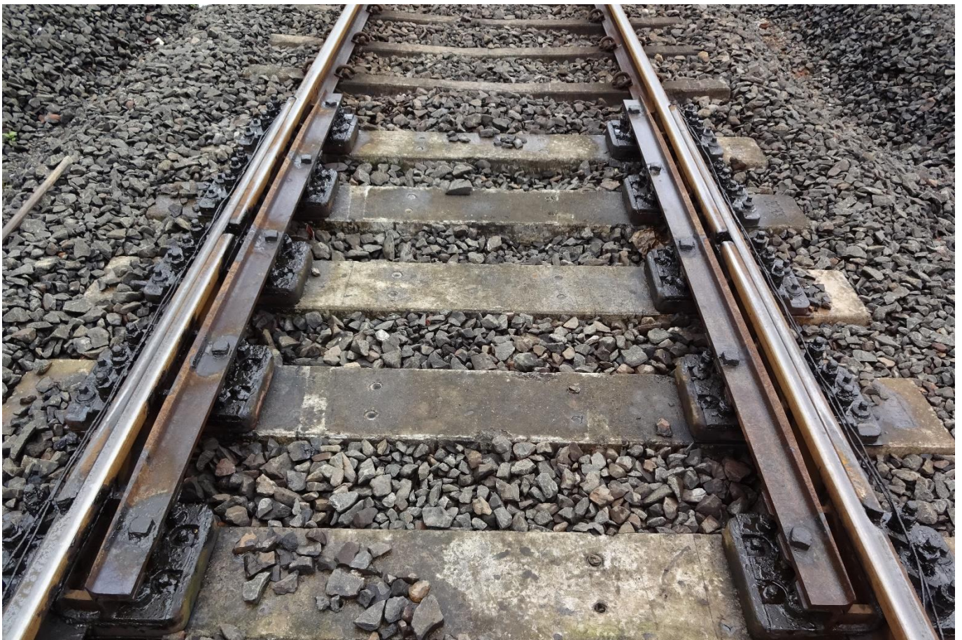
Improved Switch Expansion Joint
