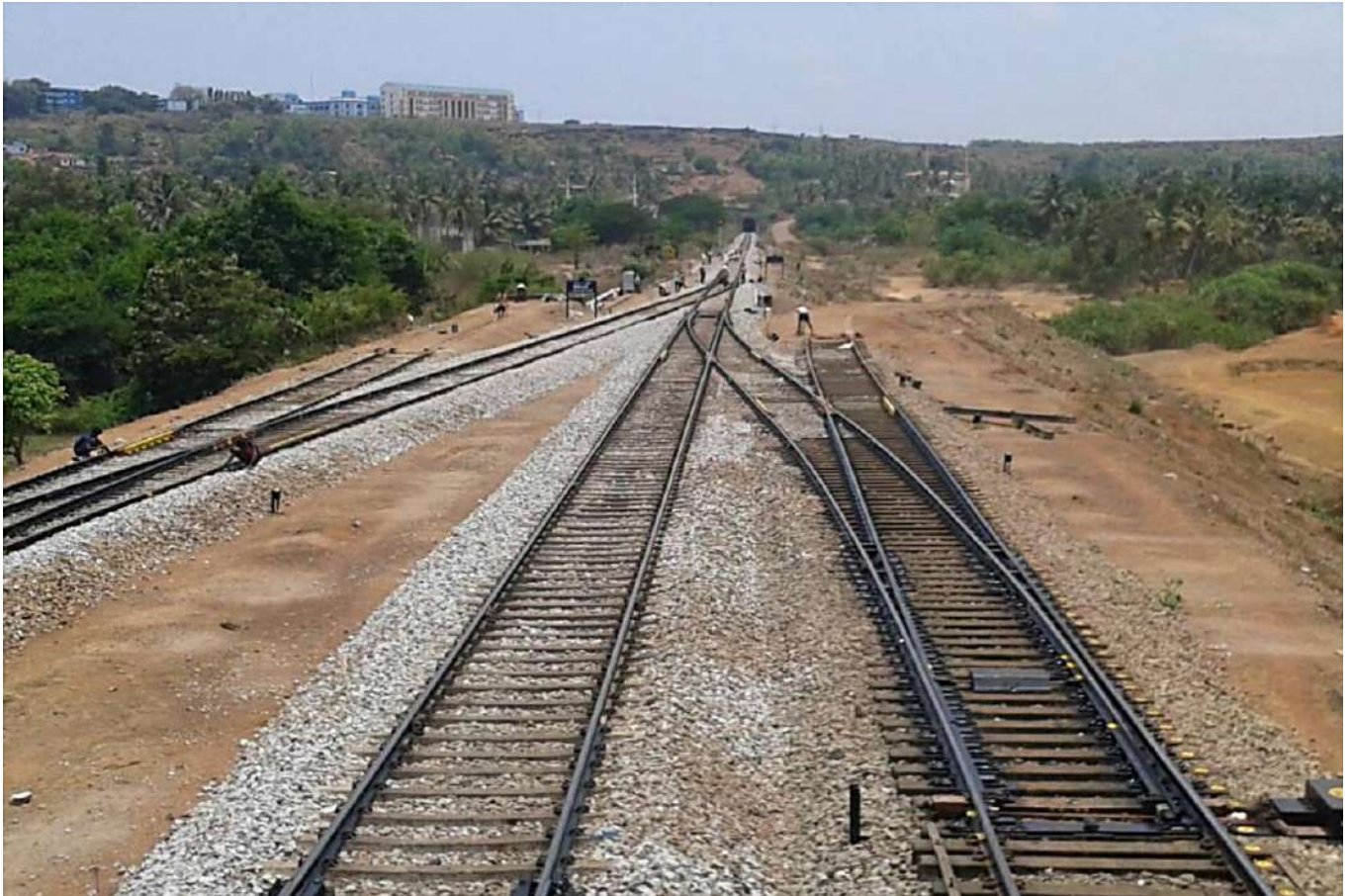
Thick Web Switches in Turn-outs
