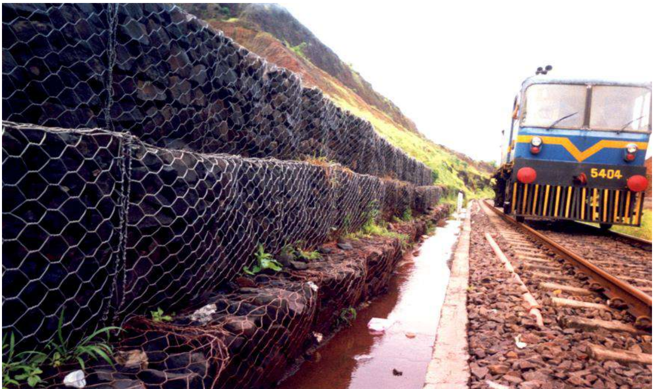
GABION RETAINING WALL
