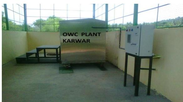
In addition "**Organic Waste Convertors**" that convert bio degradable waste into compost have been installed at Ratnagiri, Madgaon and Karwar stations. A **Bio Digester** has also been installed at Ratnagiri station's running room, and the bio gas generated is used for cooking in the kitchen. Following the success of this project, more such Organic Waste Convertors and Biodigesters are in pipeline.
